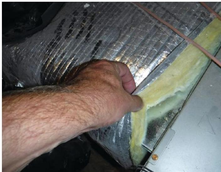
**SHORTCUTS CAUSE PROBLEMS.** Unsealed connections practically guarantee condensation when the metal surface reaches the dew point.
