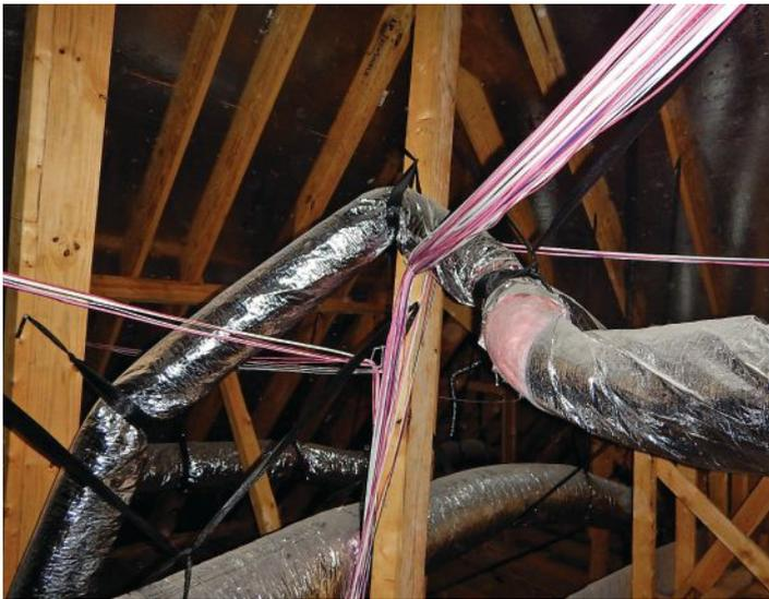
**DAMAGED VAPOR BARRIER.** The problems here include a sharp bend and straps installed to cause deep crimps. Likely consequences are insufficient airflow and condensation forming under that exposed fiberglass.
