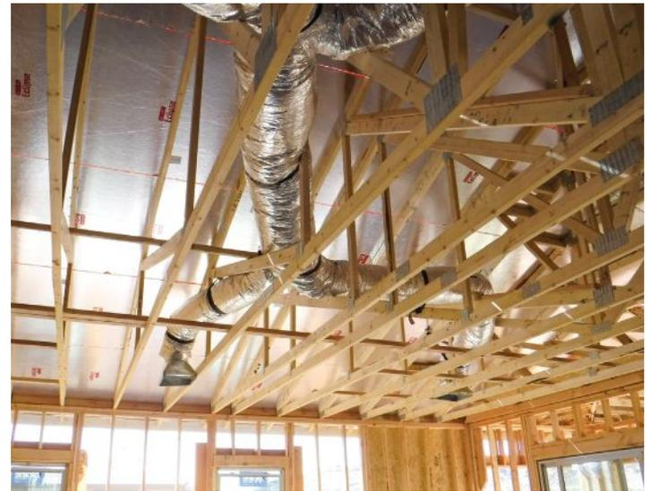
**DUCTS DONE RIGHT.** Here's an example of good practice. The duct jackets are smooth, indicating the duct has been pulled tight. Ducts are not lying on top of one another or on the truss webs. The support straps are wide enough and are spaced closely enough that they don't crimp the duct.
