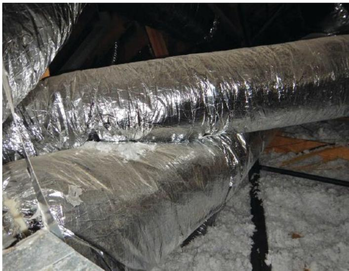
**WET SPOT.** Laying air conditioning ducts on top of one another reduces the insulation's R-value, creating a cold crack where moisture will condense. That condensation will then drip onto the attic insulation and encourage microbial growth on other building materials in the attic.
