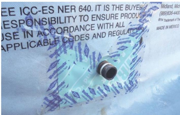
**PROPER INSTALL:** Correctly selected, flashed, and taped housewrap is critical to maintaining an effective weather barrier, especially at penetrations where moisture can easily get through.
