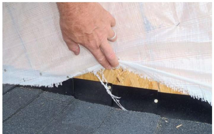
**SHREDDED EDGE:** This image illustrates how a diagonal cut in woven housewrap along a rake roof plane can quickly begin to come apart, similar to pulling a loose thread on a knitted sweater.
