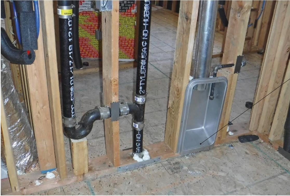
TO ELIMINATE ELBOWS, THE BASE OF THE DRYER BOX SHOULD BE AT FLOOR LEVEL, NOT RAISED ABOVE IT
