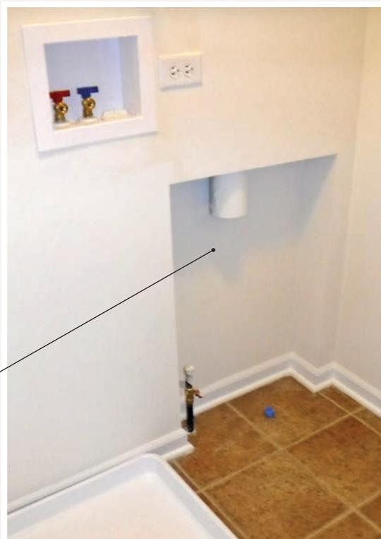
A SMALL NICHE LOOKS BETTER THAN A MANUFACTURED BOX, AND YOU NEED NOT INTERRUPT THE BASEBOARD. IT ALSO PERMITS HORIZONTAL VENTING, WHICH MANUFACTURED BOXES DO NOT
